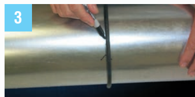
3 Use O-ring provided and mark for cut.
