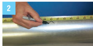
2 Mark distance to be spanned less 4".
