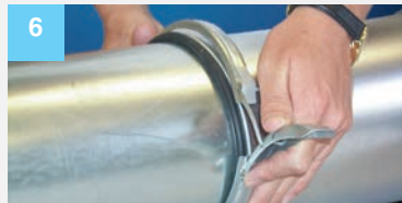
Place QF Clamp over the O-ring and end of Quick-Fit Sleeve.
