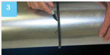
Use provided O-ring to mark for cut.
