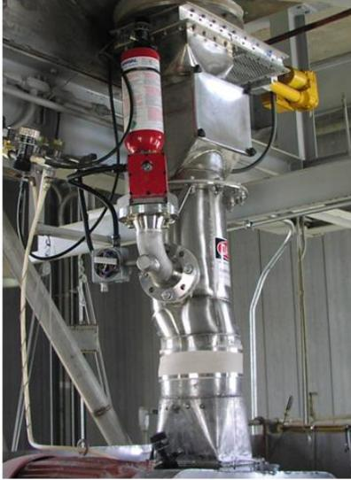
Picture 7 – Chemical isolation of a duct using a high rate discharge suppressor
