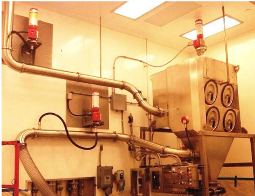
Picture 6 – Explosion protection (suppression and isolation) of an indoor dust collector
