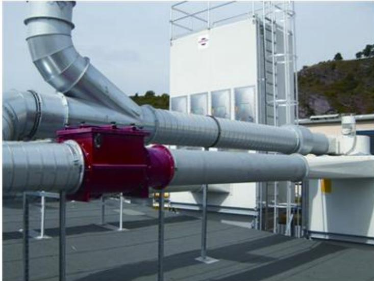
Picture 9 – Flap type valve isolating the inlet of a vented dust collector
