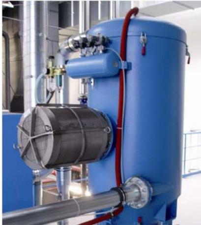
Picture 4 – Flameless vent protecting an indoor receiver
